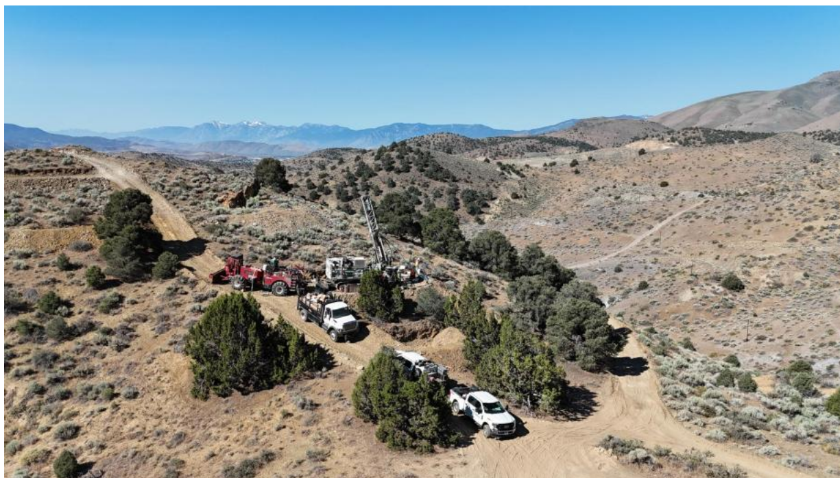
Photo 1: Drill rig assembled on site at Occidental South
